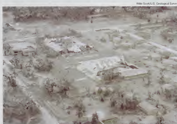
Figure 3: Buildings and vegetation at Clark Air Base, Philippines, are destroyed by a thick, wet layer of ash following the gigantic explosion of Mount Pinatubo on June 15, 1991.
